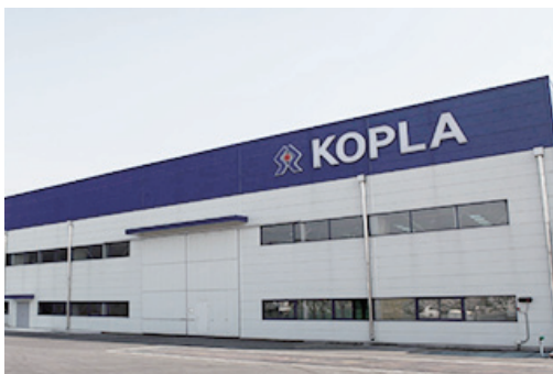
Image Courtesy of KOPLA Engineering
